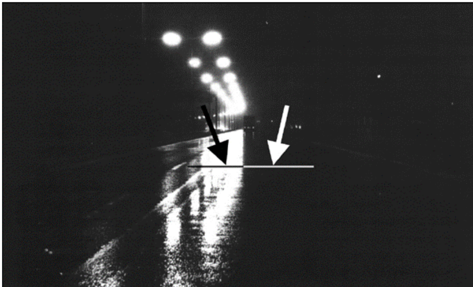
Figure 10. Different illumination of the left and right sides of the same road
